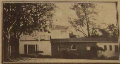
North End of Rohr Manor
