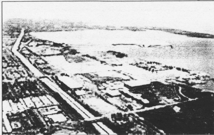
Image 2: Rohr Aircraft Industries c.1941 extending from G Street to J Street. Source: Chula Vista, the Early Years.
