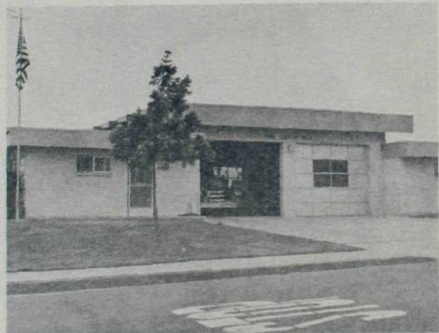
Fire Station Number Four, 5295 Otoy Lakes Road, 1965
