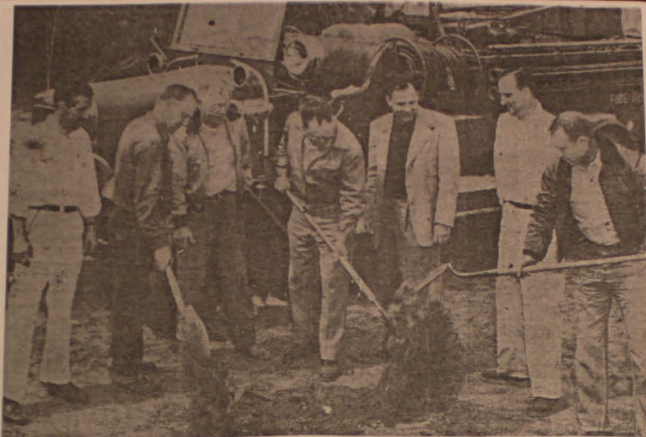
BONITA VOLUNTEERS BREAK GROUND FOR FIREHOUSE Celebrating construction of the Bonita Firehouse are, Left to Right: Bill Waters, Elmer Moore, Ralph Doughty, Dick Allen, Dick Wilson, Don Stadelle, and Scofield Bonnet.
