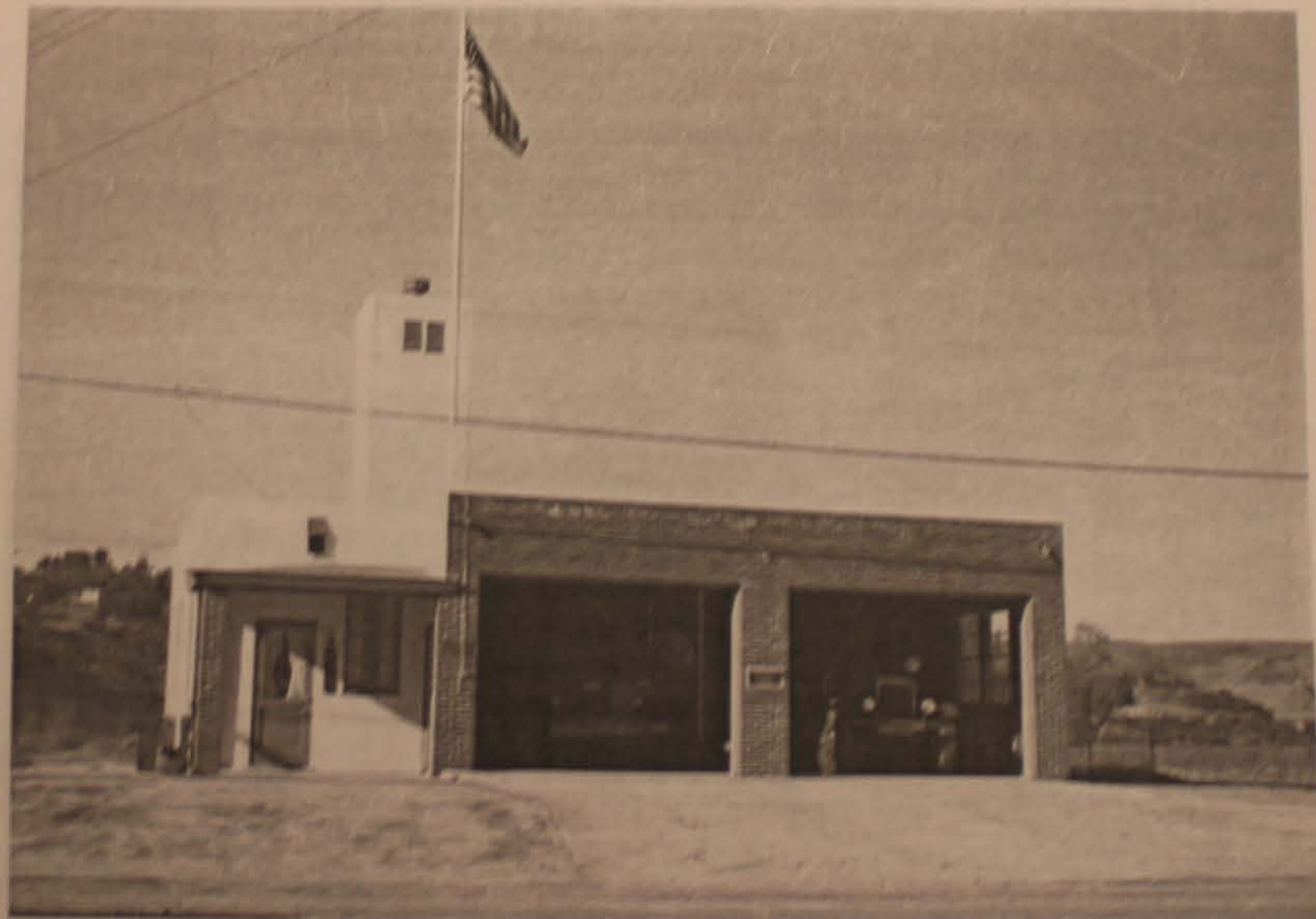
ALL MOVED IN The Upper Sweetwater Valley Volunteers are ready for the first fire out of their newly completed firehouse. Inside are one of the sprayer trucks and the 1931 Moreland.
