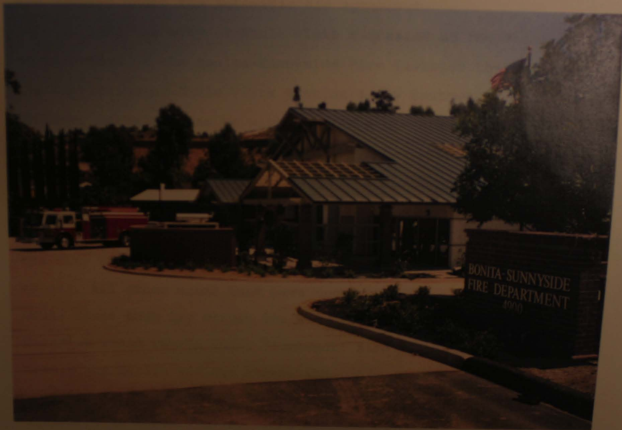
New station for the community and firefighters at 4900 Bonita Road. This, the former site of Station 2 demolished in 1991 to make way for the new station. Completed in August 1992.
