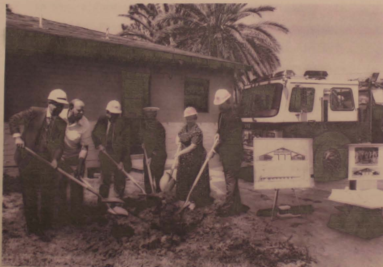
Officials celebrating the ground breaking for Bonitas new station are, James Robbins, architect; Don Ruffell, Fire Board Secretary; Tom Pocklington, Vice Chairman; Orville Moody, Fire Chief; Assemblywoman Trica Hunter; and Robert Scott, Fire District Board Chairman.
