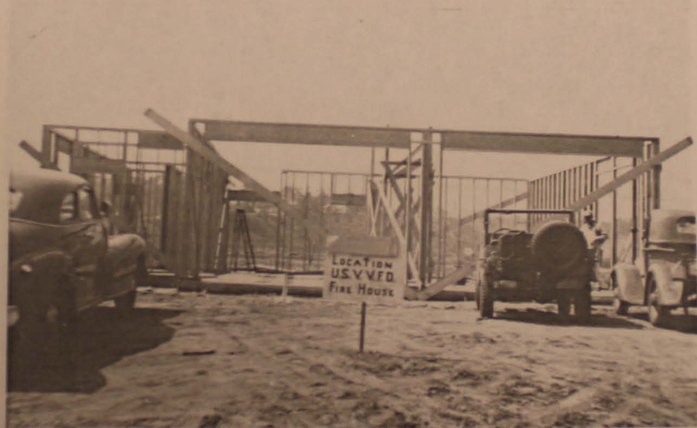
TEMPORARY SIGN IN FRONT OF FIREHOUSE Sign depicting the location of the Upper Sweetwater Valley Volunteer Fire Department during construction.
