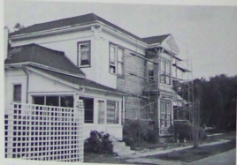
MacDonald residence 1886 644 Second during restoration
