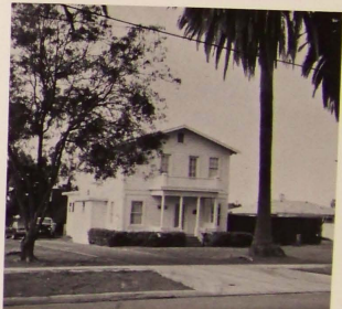
Stafford House, Historical Site No. 11, 640 Fifth Ave.
