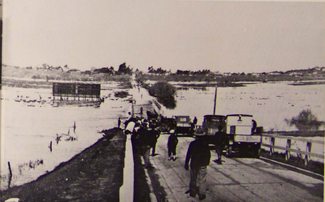
Sweetwater Dam dyke washed away and distributor sweeps through area
