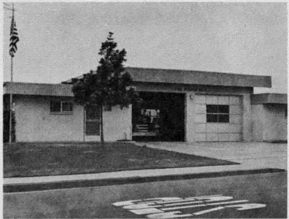
Fire Station Number Four, 5295 Otay Lakes Road, 1965
