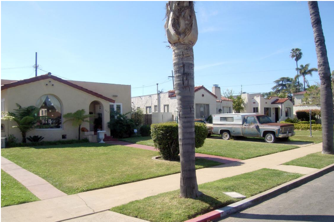
Figure 11. Streetscape view of block of Spanish Colonial Revival style single family residences, west side of 200 block of Guava.
