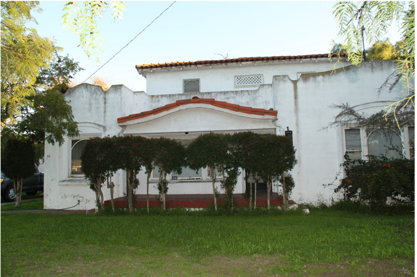
Taber Hersum house at 56 F Street
