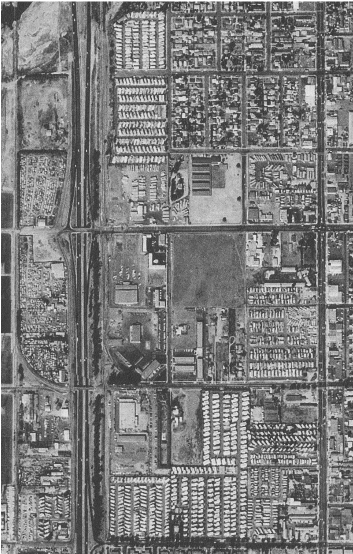
1966 aerial shows large number of trailers along G Street and at the end of D Street
